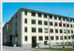
Sainte-Croix, CH heating technology
